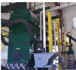
Advanced Recycling Equipment, Inc., located in St. Mary's, Pennsylvania, manufactures Challenger Biomass Combustion Systems, ranging from 1-million to 60-million BTU (240 kW to 17.6 MW). The systems are capable of burning a wide variety of biomass materials with up to 50% moisture content for energy recovery through hot air, hot water, steam, and cogeneration. Challenger thermal
