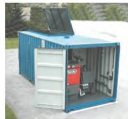
PEI-based Wood4heating offers contract heat provided from Austrian Binder biomass boilers fired by wood chips, pellets, or other biomass. Ranging from 150 kW hot water to 10 MW hot water or steam, the customer pays only for the BTU/kWh consumed based on biomass input. Wood4heating sizes and purchases the boiler, installs and runs it, and procures the fuel, providing heat to the customer
