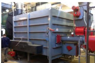
Chiptec Corp. produces Chiptec Wood Energy Systems. These fixed-grate, close-coupled gasifier systems range from 300 kW to 20 MW thermal output. Cogeneration capacity is available at 300 to 900 psig. The gasifiers can fire almost all boiler types, from low-
