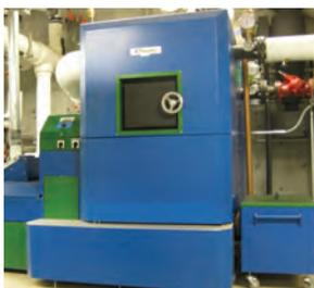
ACT Bioenergy manufactures high-efficiency biomass boilers ranging from 150 to 500 kW thermal. Our underfed grate, gasification-type hot water boilers are user-friendly, with automated ignition, feed control, and ash removal. High efficiency and exceptionally low emissions are achieved by constant monitoring of combustion chamber temperatures, oxygen levels, and pressures, and automatic
