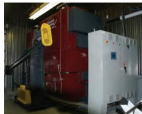
Transfab offers systems of 400 kW and greater thermal output and can burn wood residues, chips, pellets, and even bark with up to 60% moisture content. The company manufactures fixed or mobile grate (step or flat) furnaces that burn a large range of dry or wet biomass. It specializes in ASME low- or high-pressure fire-tube boilers (HRT, dryback, wetback,
