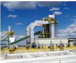
Deltech offers biomass boilers in the range of 500 kW to 50 MW (1.7-million to 170-million BTU/hour) thermal output, with available cogeneration capacity typically 0.2 to 5 MW electrical. Furnaces are pile, pellet fixed-bed, or step-grate burners, heating low-pressure hot water or thermal oil boilers. Applications include sawmills, wood
