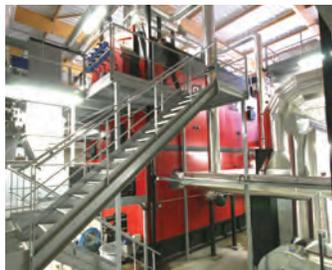
Compte-Fournier is the biomass boiler technology supplying renewable energy to the London 2012 Olympic Games. Compte-Fournier offers fully automated, high-efficiency biomass boilers with Compte-R technology in North America. Hot water boilers range from 250 kW to 10 MW, steam boilers have output of 2 to 12 t/h at pressure
