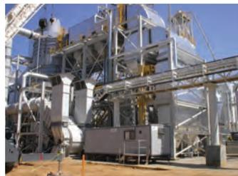
EPI's fluidized bed boiler systems convert renewable biomass and other solid or liquid fuels into steam energy and range from 5 to 60 MW thermal output. From major superheated utility power boilers to small heat recovery boilers, EPI systems feature a state-of-the-art fluidized bed thermal oxidizer combined with advanced
