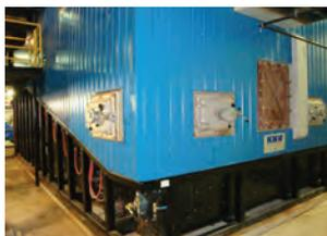
KMW Energy Inc. offers heat energy only or combined heat and power (CHP) plants complete with power generating equipment. Thermal-only systems range from 150 boiler hp (1.5 MW thermal) to over 4,000 boiler hp (40 MW thermal); CHP plants range from 1 to 25 MW electric.
